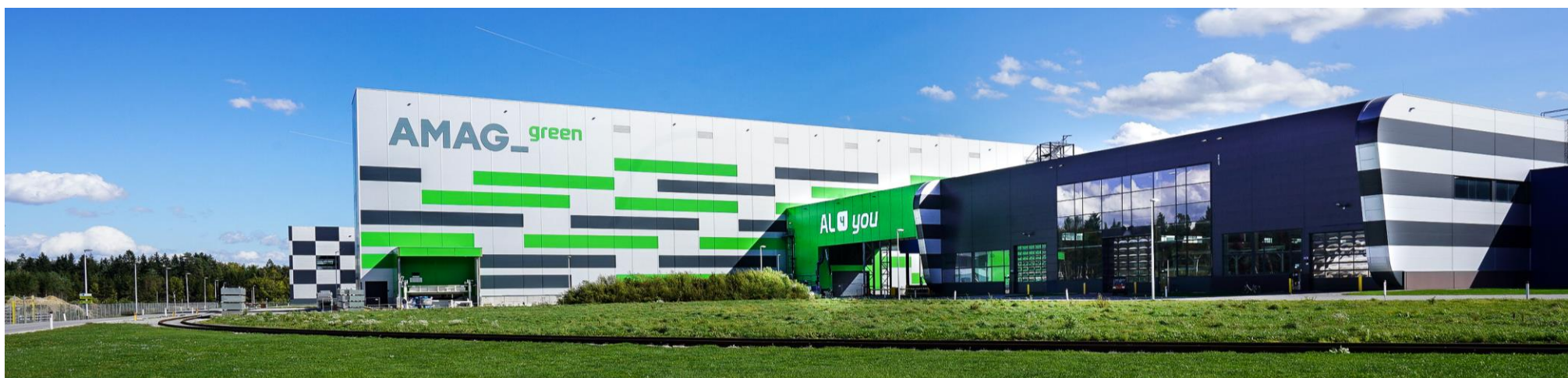
The new rolling slab high-bay warehouse
