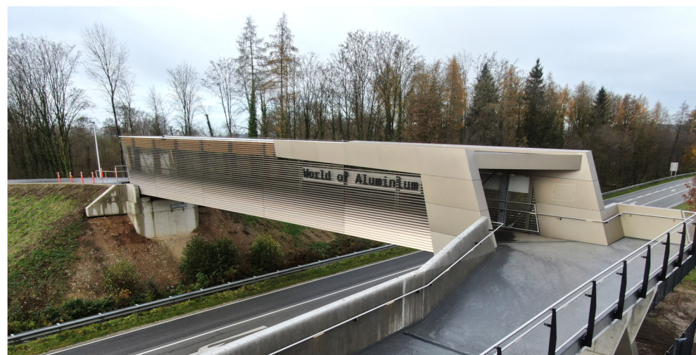
Investment in occupational safety: Award-winning “Cycle and Pedestrian Crossing”, constructed with wood from the AMAG forest
