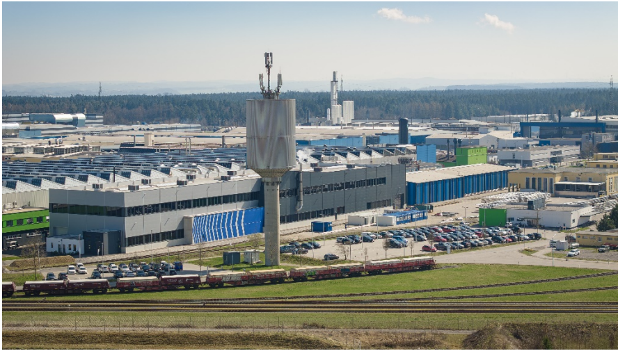
Image 3: The 115-metre-long plant is located in a building that was constructed by regional suppliers. (©AMAG)
