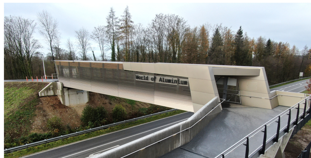
Investment in occupational safety: Award-winning "Cycle and Pedestrian Crossing", constructed with wood from the AMAG forest
